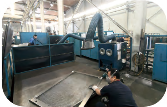
Efficient ventilation equipment and appropriate labor supplies are installed and provided in the welding process
