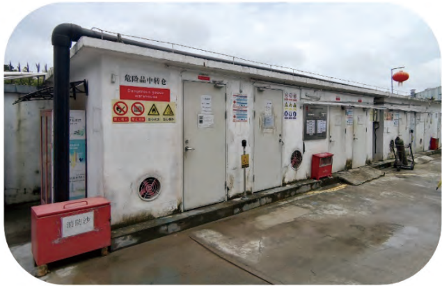
Hazardous Waste Warehouses in Shenzhen plant
